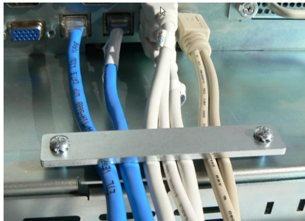
Cable Securing Bar Installed
